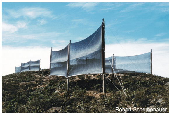
A portion of the array of large fog collectors at El Tofo, Chile. The distance between posts is 12 meters.
